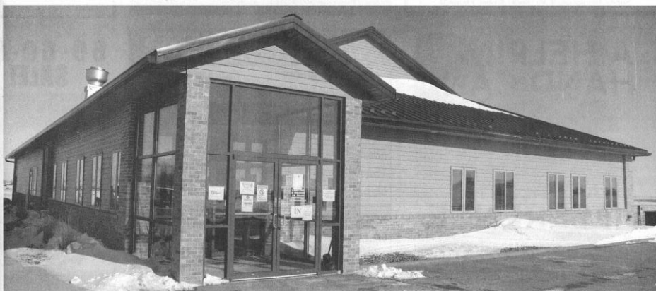
New Opportunities opened its Early Head Start Center at 1617 E. 10th St. in January. The building formerly housed various businesses and was renovated to include four classrooms for infants to 3-year-olds.
